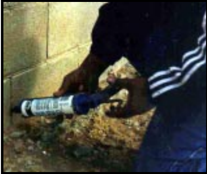
Seal holes with caulk
