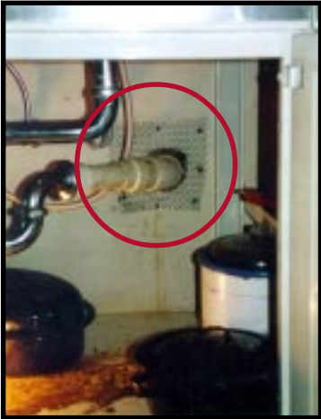
Use lath metal around pipes
